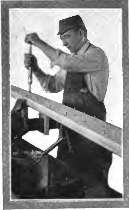
Fig. 3—Screwing the laminations of the sill together
